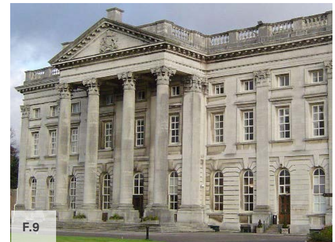
Figure 09: Moor Park and orangery, grade I listed building.
